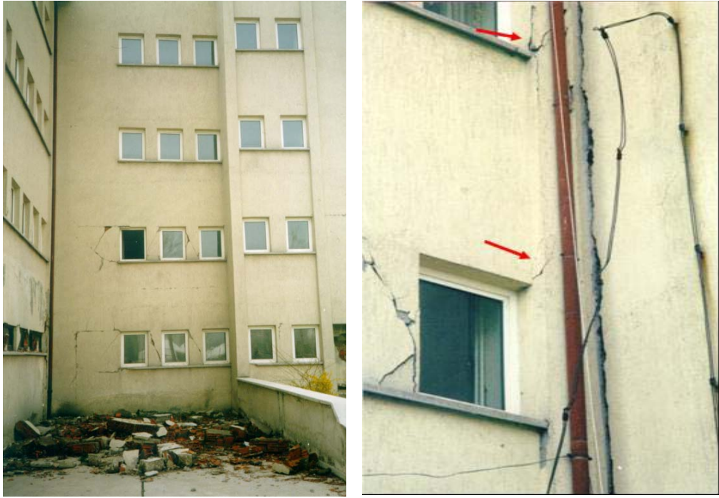
Figure 5. Close-up View of Building Joint in Bolu
