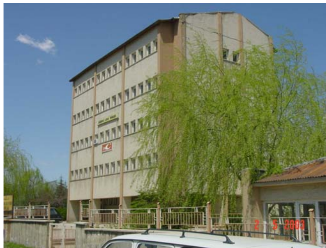
Figure 2. MPWS Branch Building in Bingöl
