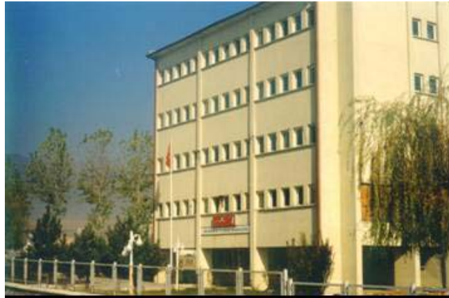
Figure 1. MPWS Branch Building in Bolu
